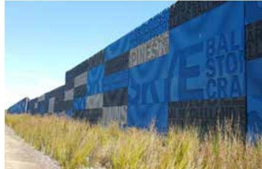
With construction of the M5 Freeway in New South Wales, Qenos provided Alkatuff® LL711UV polymer for the sound wall panels to be rotomoulded by Viscount into 6 m lengths, up to 600 mm high and 30 mm deep, with a UV requirement of 18 years. Over nine months, 15,000 individual panels were installed across 18 km.
